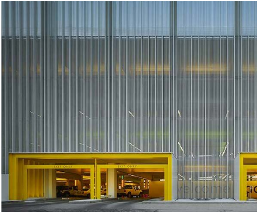
Chesapeake Car Park 4, Rand Elliot Architects
